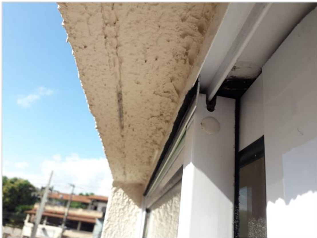
Figure 19 – Solution employed for sealing of main crevice
